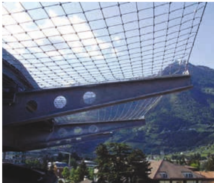
Dralo® used to secure the edges of a helicopter landing pad at a hospital in Meran.
