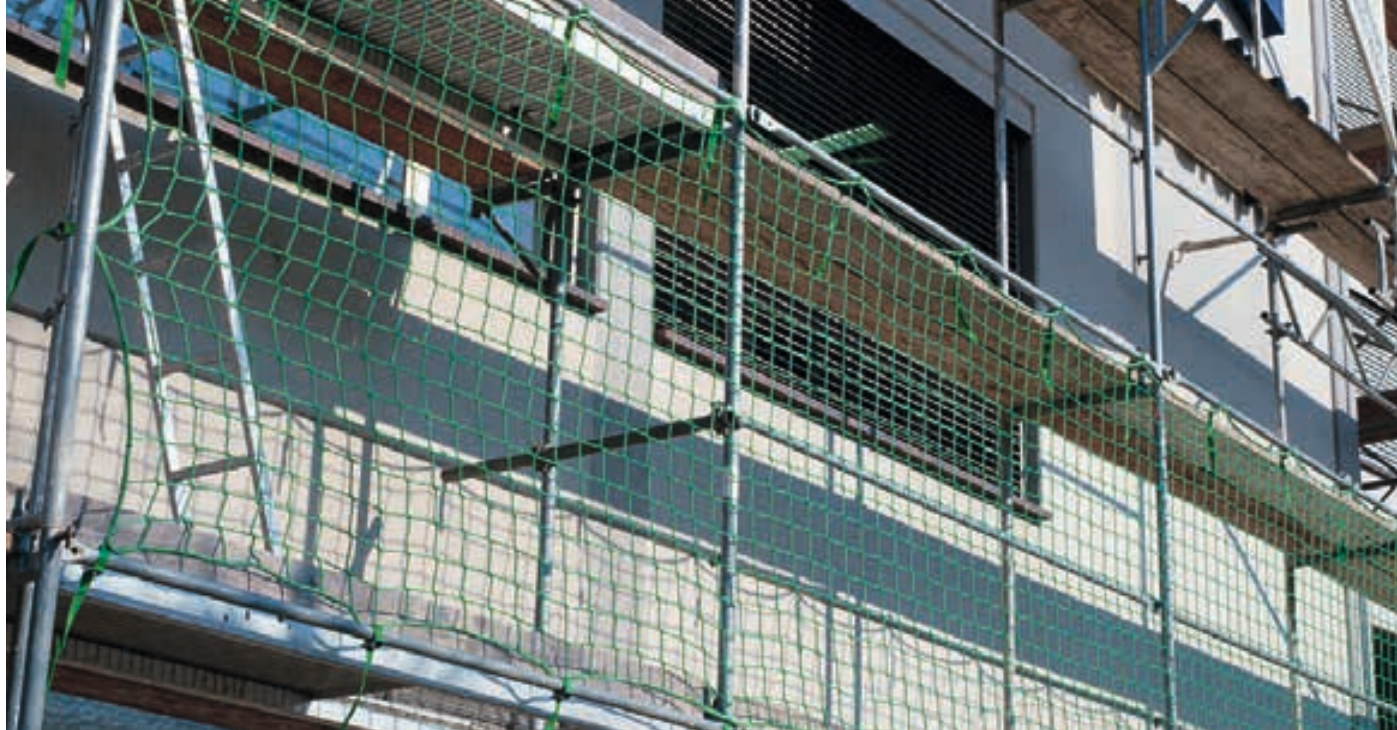
Brick guardrail net, mesh size 100 mm.
