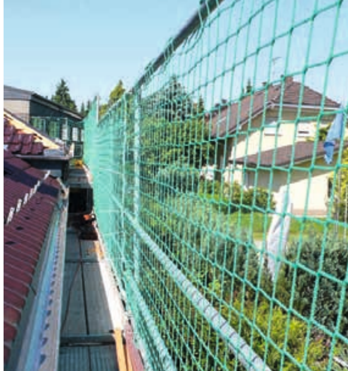
The guardrail is secured to the load-bearing construction mesh.
