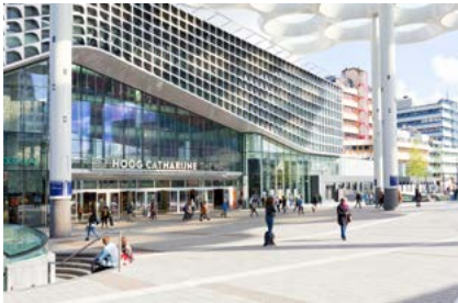
Parking Garage Hoog Catharijne - Utrecht the Netherlands
