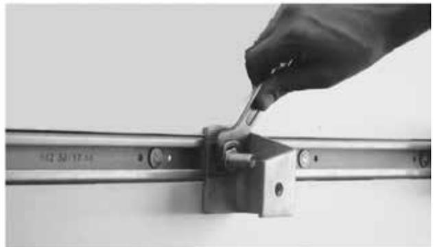
4.) Fixtures are fastened with the T bolts and nuts as shown above. Correct loading and torque values need to be applied in accordance with the allowable loads of the channels and bolts.
