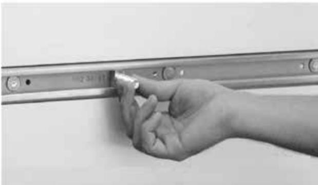
3.) Connections to the cast in channels are made with T bolts and lock nuts. T bolts are inserted in to the channels horizontally and then turned right through 90 degrees. This locks them vertically in the channel.
