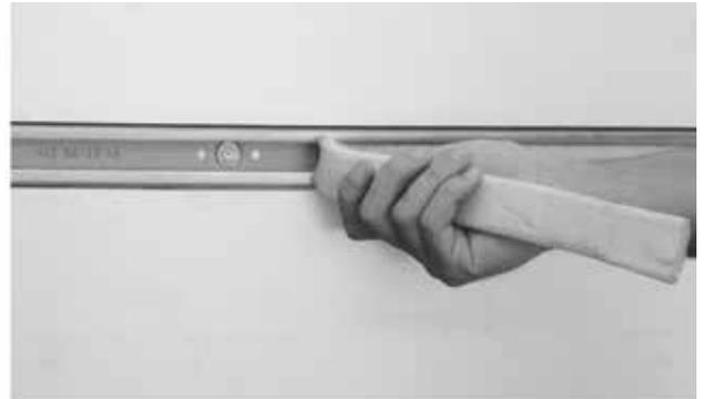
2.) After the concrete is cured, the filler inside the channel, set for the purpose of preventing concrete filling the channel's slot, is removed as shown.
