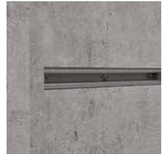
4.) No filler or concrete left overs should be left within the channel slot. Any residue should be scrapped out
