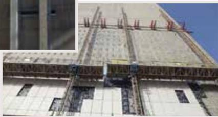
*Curtain wall cladding fixed on anchor channels on the edge of slab*
