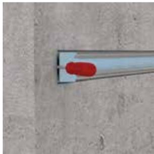
2.) After concrete has dried out, the filler in the channel should be taken out using a suitable tool
